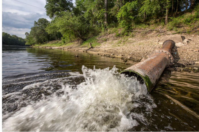
In Live Oak, Florida, wastewater pours from a Pilgrim's Pride meat processing plant into the Suwannee River
